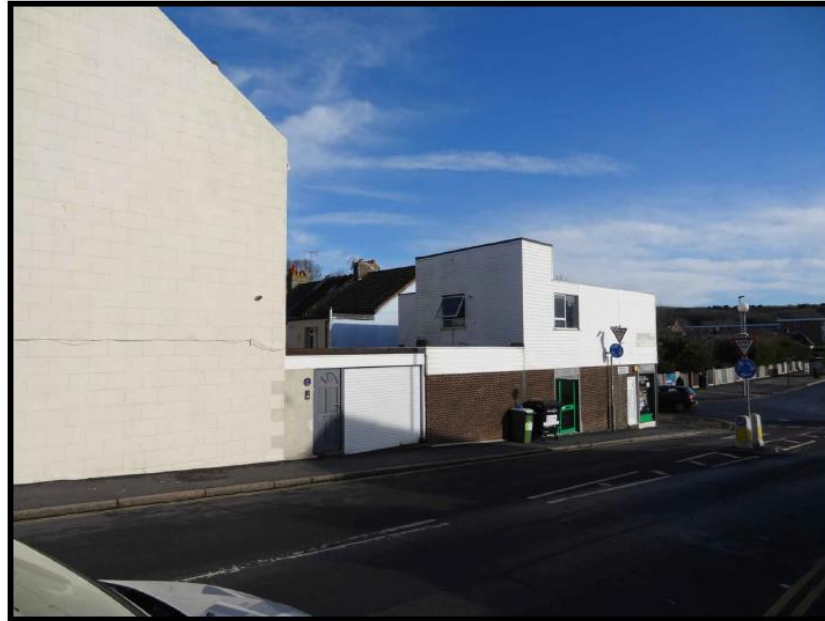
Photo of Site as Existing (South West View)
